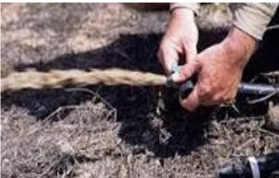
Figure 10.7: Flushing the lateral.
