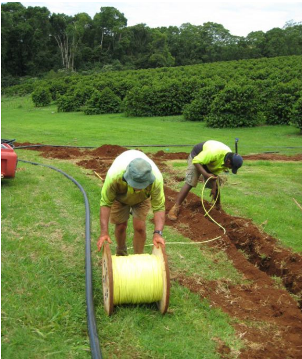
Figure 6.8: Laying electric conduit and irrigation pipes in new trenches.
