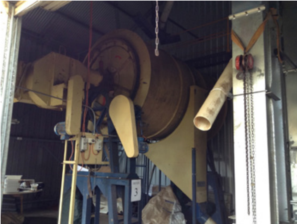
Mechanical drying equipment
